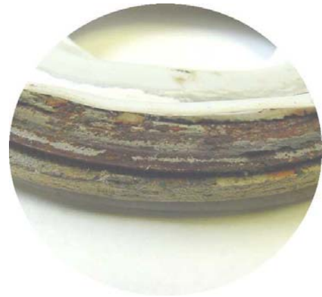
Cross-section of a chemically attacked envelope gasket with a non-asbestos filler
