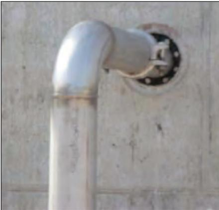
Many of these applications involve connections where the pipe is penetrating a wall, floor or ceiling and sealability is required between the pipe and the penetrated surface. Through wall applications are an area where a mechanical seal needs to be utilized in order to reach complete sealability.
